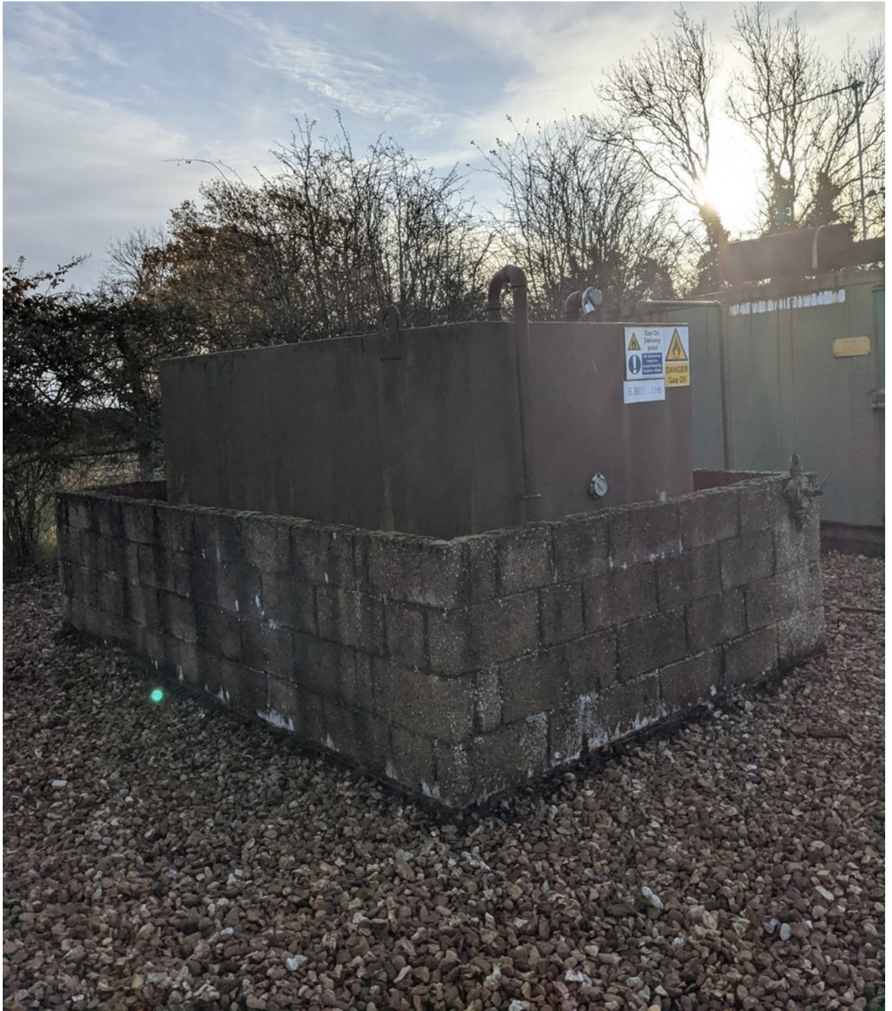
Photo 1: Waterbeach WRC fuel tank
